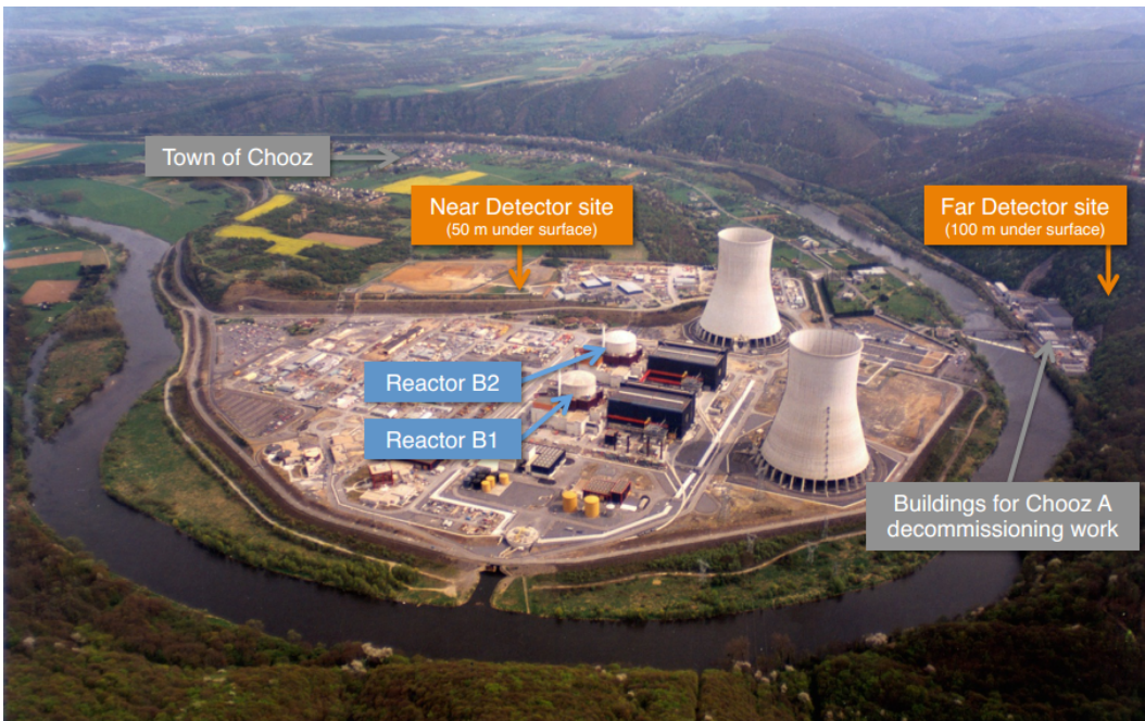
Figure 3.7: Overview of the DC site indicating the location of B1 and B2 reactors and the ND and FD, from [69].
