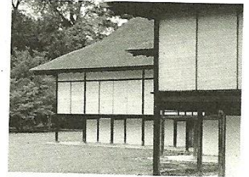
1620 Katsura Detached Palace, Kyoto: raised on pilotis.
